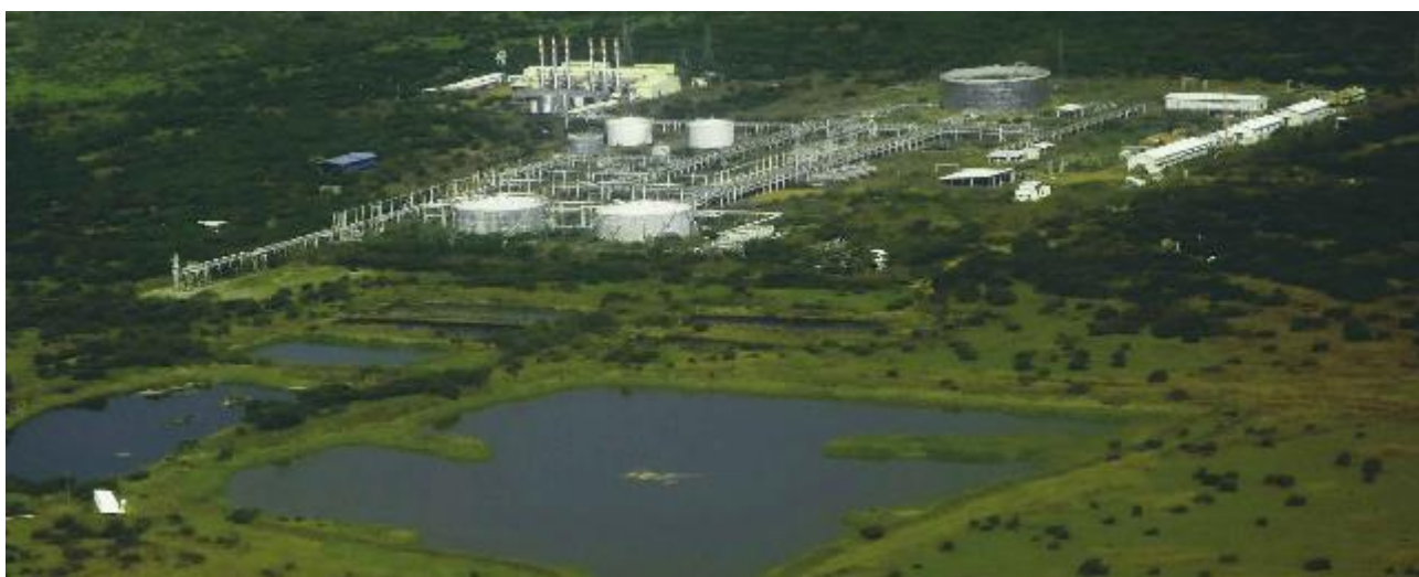
Produced water ponds along Paloch Oil Field. Credit: Department of Health Safety and Environment (HSE), South Sudan Petroleum Authority, Ministry of Petroleum
