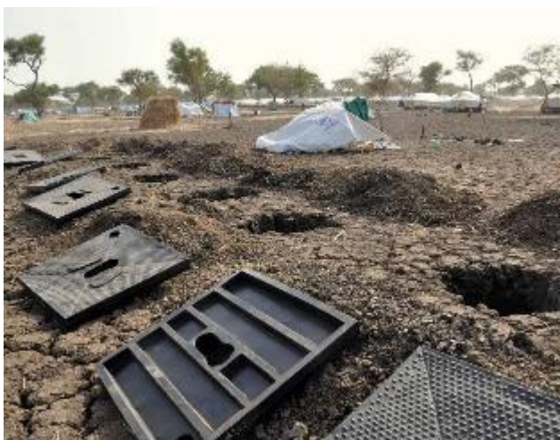
Latrine slabs waiting to be installed, Jamam refugee camp.
