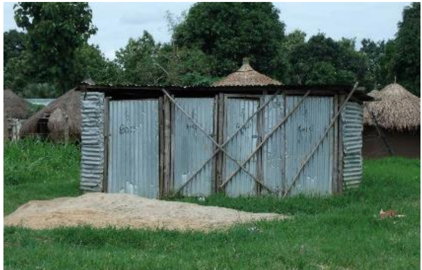
Pit toilet with super structure built in metal sheets.
